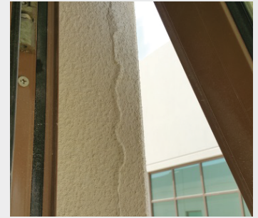
HAIRLINE CRACKING
