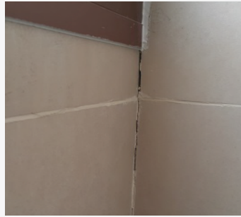
MISSING GROUTING
